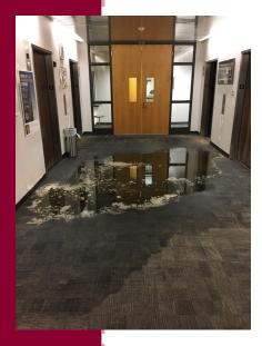
In mid-November, the Department of Commerce and Division of Real Estate employees arrived at work to find significant flooding and water damage throughout the Heber M. Wells Building as a result of ruptured ceiling water pipes. Water intrusion throughout the building and down elevator shafts required extensive repair work to office spaces and retrofit work to restore elevator service. In late April all water damage repairs had been completed and elevator service was restored.
